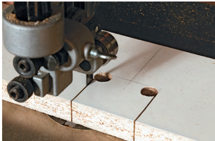
Cut out the opening after drilling at the corners. Freehand cuts at the bandsaw make quick work of the opening. Drilling at the corners lets you navigate the turn with the bandsaw blade much more easily.
